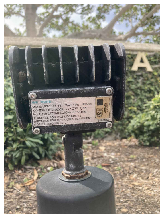
EXISTING CORNER SIGNAGE UPLIGHT (6 TOTAL)
